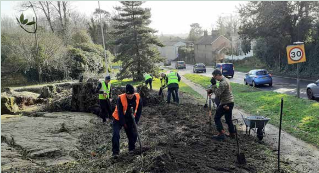
Volunteers clearance work at The Rusthall Spring Site
